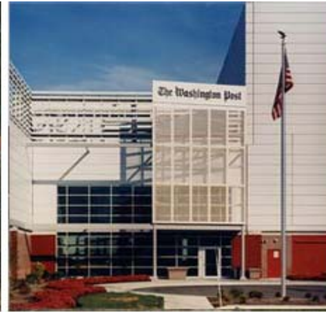
The Washington Post Printing Plant - Washington DC
